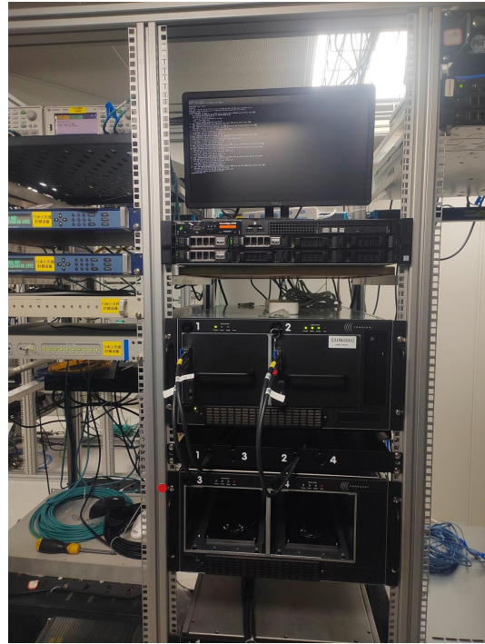
Fig. 3 MK6 recording system in the EM-shielded basement at the Urumqi station.
