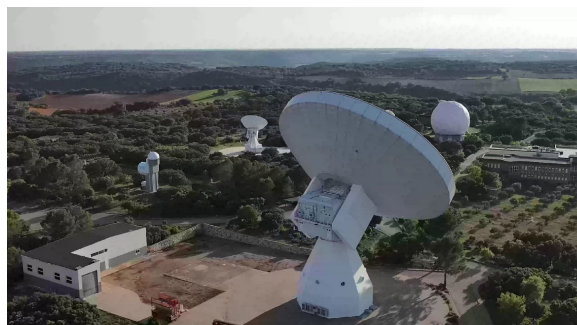
Fig. 1 General view of Yebes Observatory.
