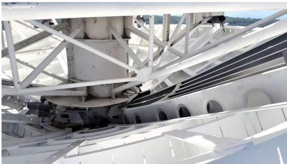
Fig. 5 Panel replacement process (one panel left to replace).
