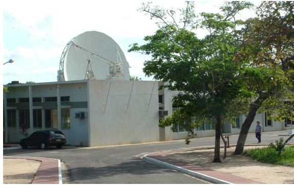
Main building with the VLBI antenna in the background.
