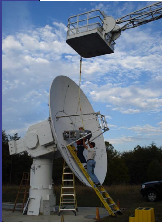
Jay Redmond and Bruce Whittier installing the Dewar on the 5m MV-3 antenna.
