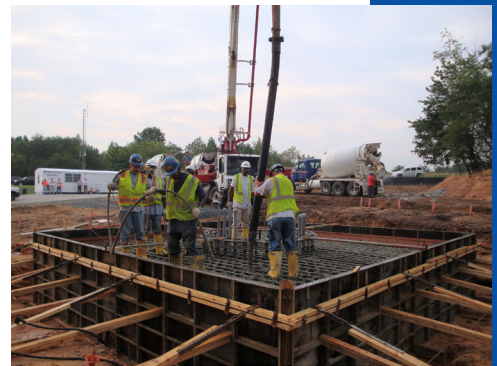
(top) 25 auger cast pilings were bored before 61 cubic meters of concrete were added in a continuous pour to complete the 12 meter VLBI2010 antenna foundation. (below) Irv Diegel, of Honeywell Technology Solutions, Inc., works to integrate temperature control electronics into a prototype broadband phase calibrator.
