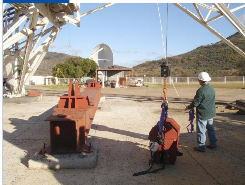
Darren Forren (GD Satcom) prepares to lift the universal knuckle joint that will join the A-frame legs to the polar shaft support collar. The 15-m single piece fiber-glass composite prototype KAT antenna is visible in the background.
