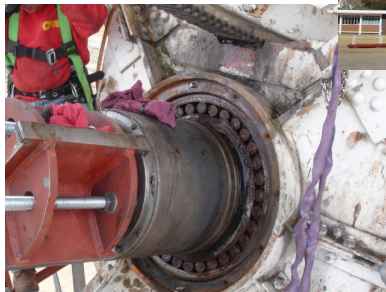
(left) With the antenna safely supported, the top end of the fixed part of the polar shaft has now been removed to expose the failed bearing. Damage to the inner race is clearly visible on the right. (top) The Hartbeesthoek 26-m antenna drives over to the west for the first time following the replacement of the south polar shaft bearing.
