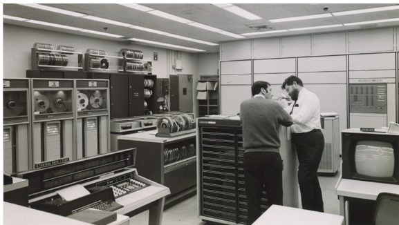
(left) CDC 3300 computer at Haystack Observatory; correlated and processed VLBI experiments 1967-1969; (right) VLBI front end for OVRO 90' antenna for October 1969 experiment; nested L-band/X-band feeds.
