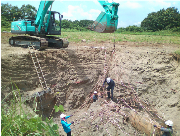
Excavation work for the antenna foundation at the Ishioka site.
