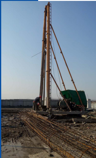
Construction work at the Sheshan VGOS site.
