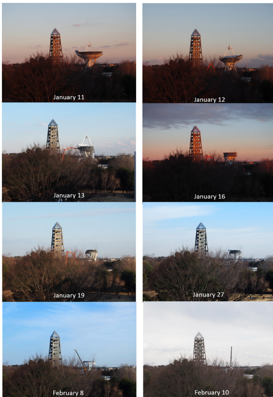
Progress of the dismantling of Tsukuba from January 11 through February 10.
