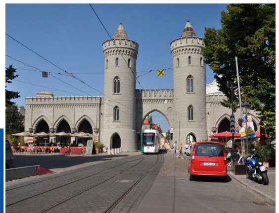
The Nauener Tor (Nauen Gate) is one of the three preserved gates of Potsdam. Today a tram line leads directly through the gate.
