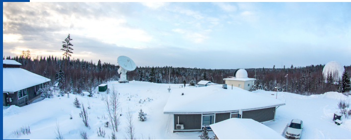
Panorama of Metsähovi (from the left): the gravimetric laboratory, VGOS telescope, main building, new SLR dome, and the radome of Aalto University radio telescope. (Photo Jyri Näränen)
