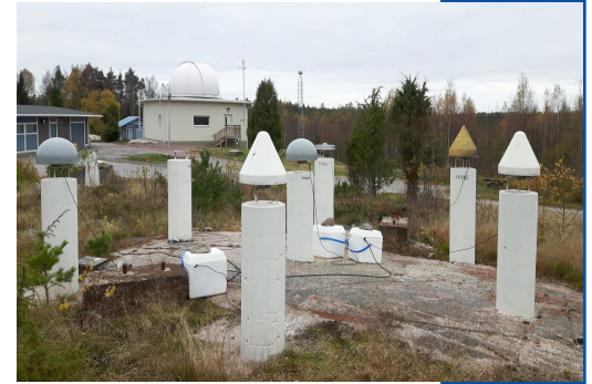
GNSS antenna test field. The new SLR dome is in the background.
