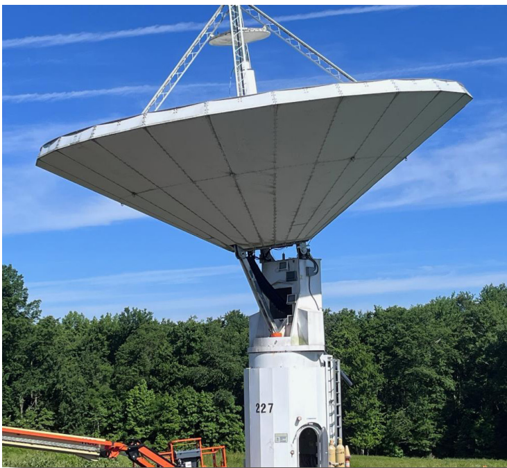
GGAO 12-m antenna with the new jackscrew.
