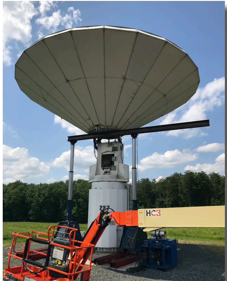
GGAO 12-m antenna following removal of the old jackscrew.
