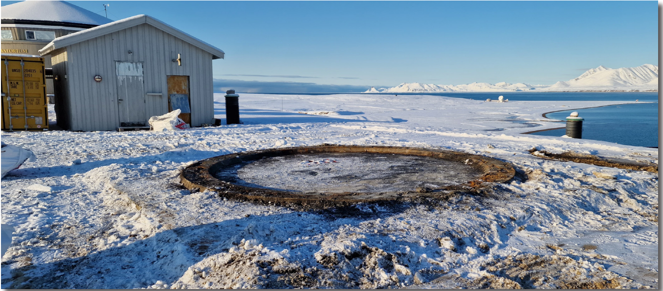
The site of the former Ny antenna after dismantling. In the distance (about 1.5 km) the new Brandal Geodetic Observatory with the Nn and Ns antennas.
