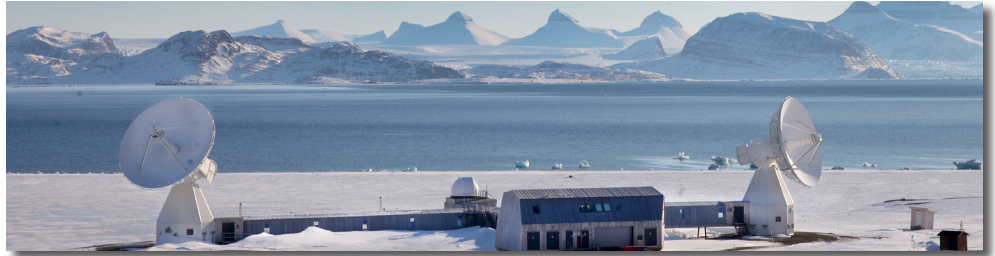
The Geodetic Observatory featured a 20-meter legacy S/X VLBI radio telescope at the Rabben site until August 2023 (left), as well as fast-slewing VGOS twin telescopes at the new facility at Brandal Geodetic Observatory (right).
