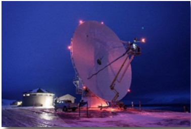
The Geodetic Observatory featured a 20-meter legacy S/X VLBI radio telescope at the Rabben site until August 2023 (left), as well as fast-slewing VGOS twin telescopes at the new facility at Brandal Geodetic Observatory (right).
