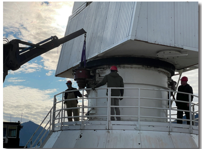
Our colleagues from GBO working on the 20-m antenna, taking panels and gear boxes as spare parts.
