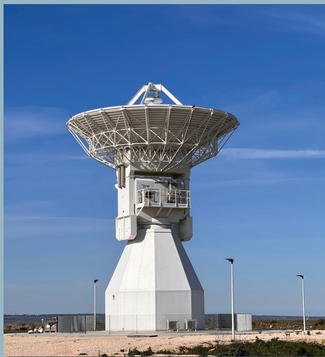
The new Matera VGOS antenna at the ASI Space Centre. Avanti VGOS!
